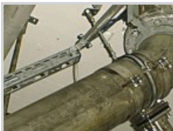
MARTIN® PKL® Interval Impactor on transfer pipe
